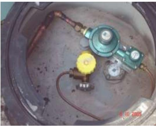
LPG Regulator type as determined by the Gas fitter) and Pig Tail
